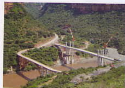
Old Abai Bridge (Left) and Hedase Bridge (Right)
