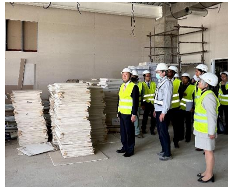
Visit to construction site
